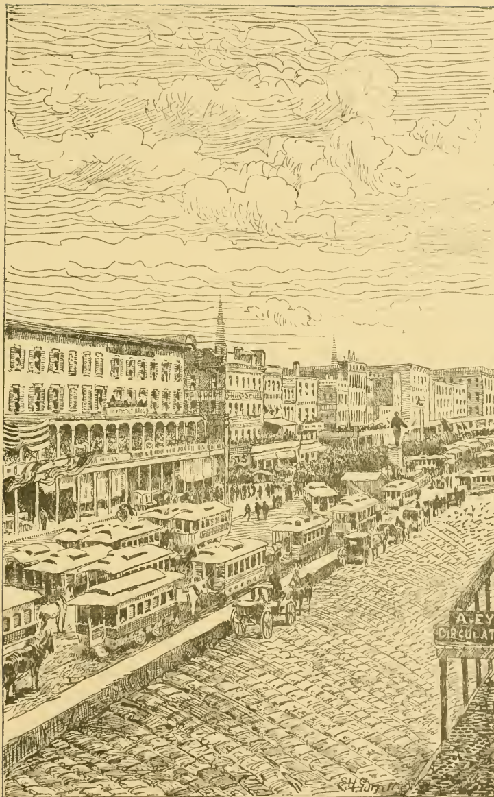
CANAL STREET, NEW ORLEANS.
